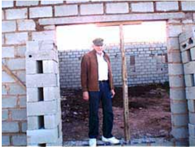
Jim in the half-built hospital. The far wall is the one that fell, killing two students.
